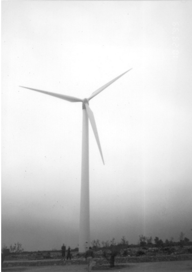
Figure 10.6 750 kW wind turbine from the Parc Eolic de Colladeres, Spain
