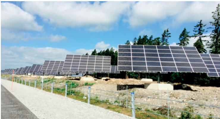
Figure 2.3. A park of solar-tracking PV arrays in Västerås, Sweden. Photo: Joakim Munkhammar 2014.
