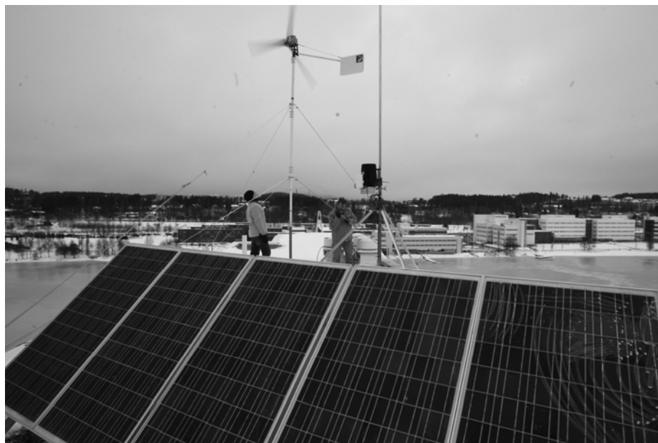
Figure 11. PV panel array (100 W each), wind turbine (500 W) and a weather station at the roof of the physical chemistry building of the University of Jyväskylä, Finland. (photo: RE program)
