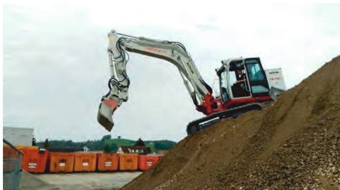
Figure 9: 16 t electric excavator deployed on a building site (Source: www.suncar-hk.com )
