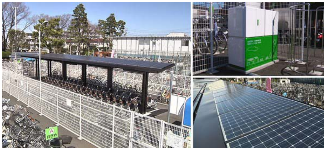
Figure 66: Sanyo solar powered charging station in Tokyo, located at the train station.
