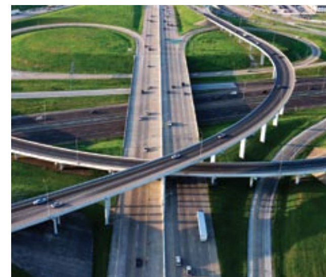
An aerial view of a clover leaf interchange on the U.S. interstate highways.
