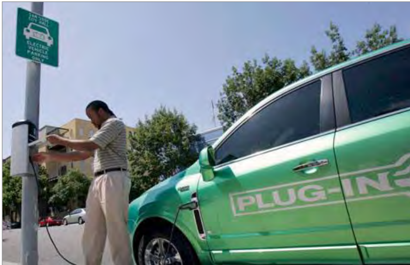
Figure 4-2: Public charging facilities, California
